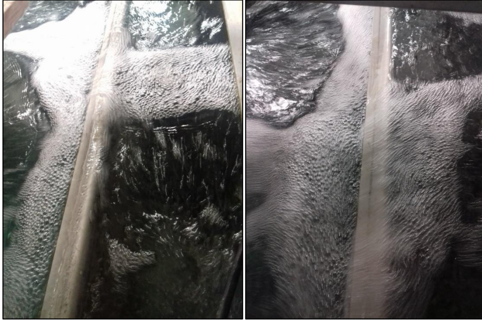
Figure 5.12 Backflow between Basins 3 and 2 due to Aeration
