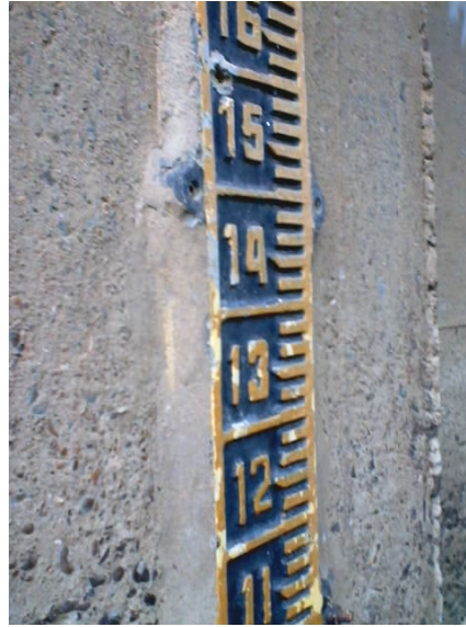
Photo 3.1. Level marker attached to a bridge's pile
