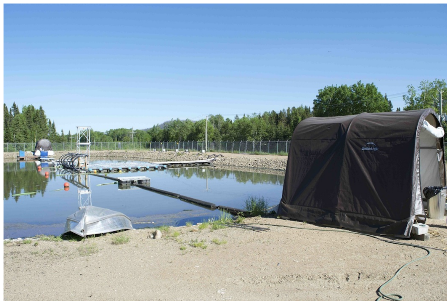
Figure 1: The first lagoon in Wemotaci. In the brown tent on the right is the first monEAU station installed at the inlet of the lagoon and on the other side is the second monEAU station installed at the outlet of the lagoon. In between are the bio-reactors of Bionest installed.
