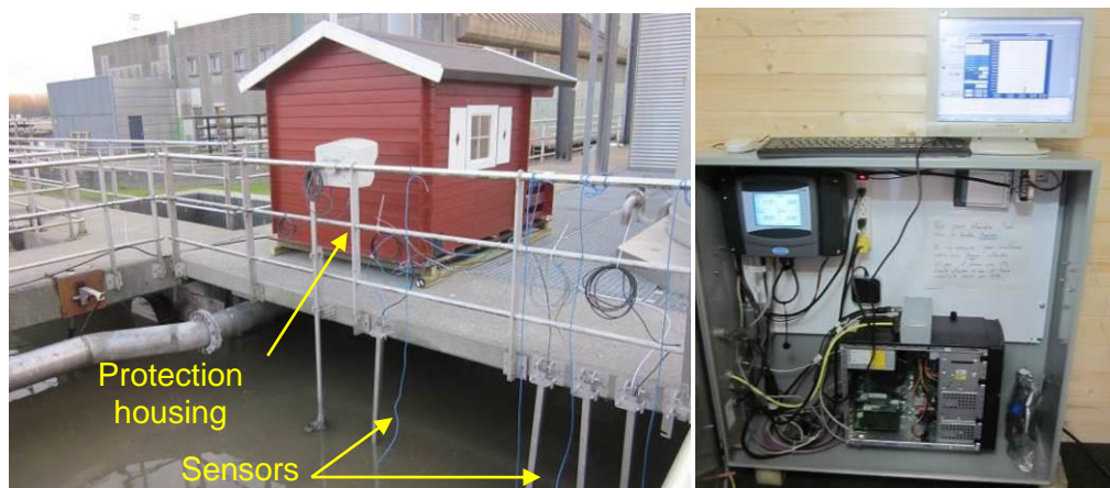
Figure 1. Installation of monitoring station: Housing (left); RSM30 monitoring station (right)
