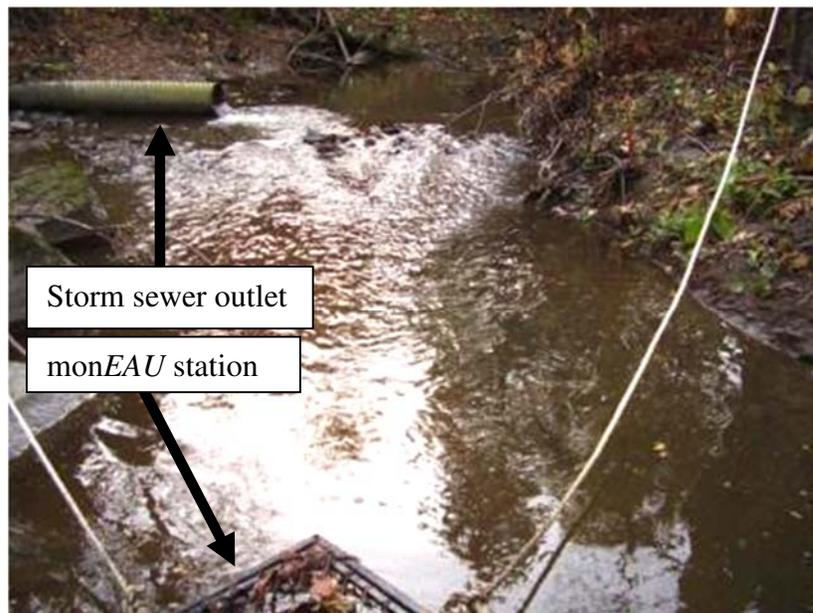
Figure 63 : Storm sewer outlet just upstream the monEAU station
