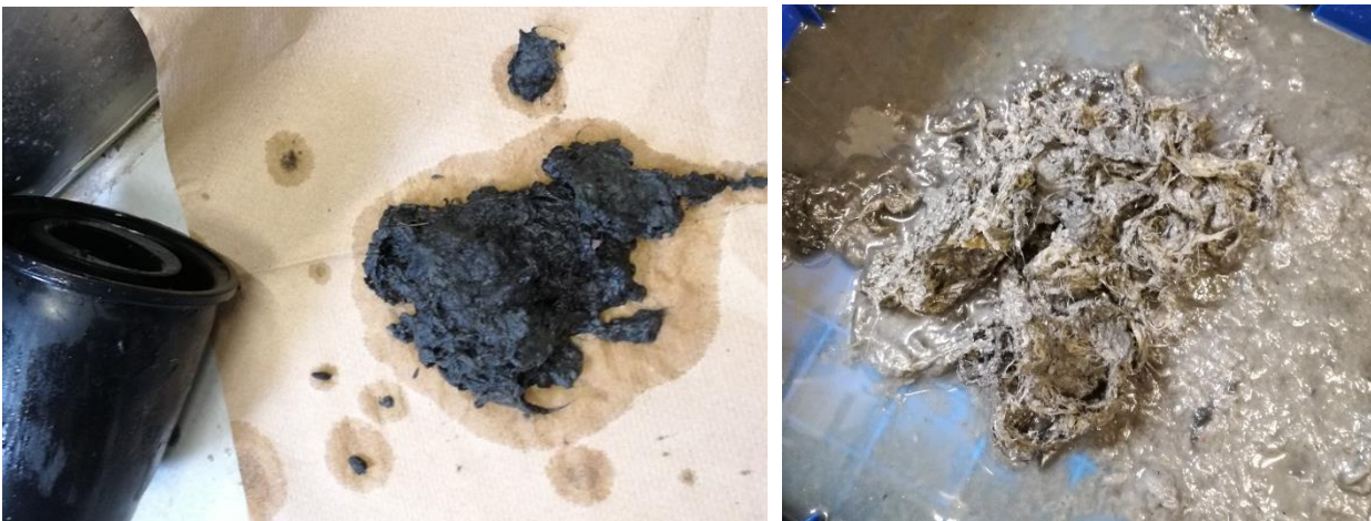
Figure 45: Materials found in the recirculation line pump causing the clogging.
