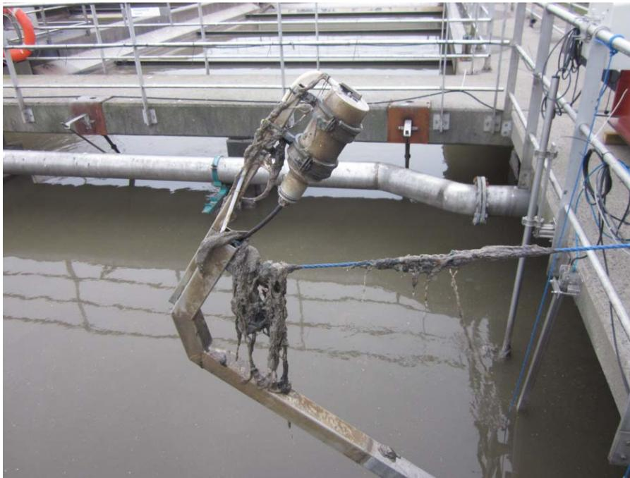
**Figure 6 – The case study turbidity sensor – Sensor fouling problems**
