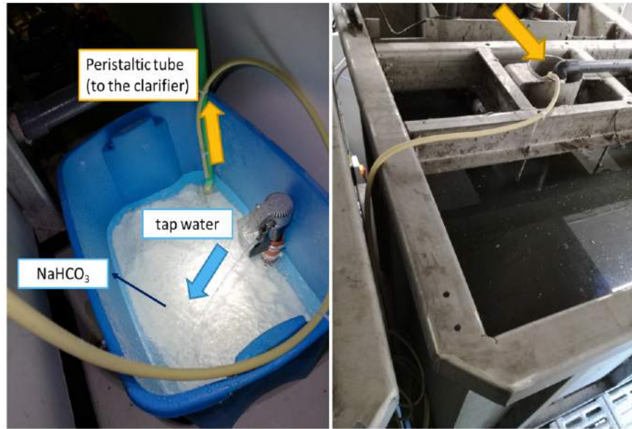
Figure 4.27: Alkalinity dosing set-up at the pilEAUte using a saturated sodium bicarbonate solution. Left: the dosing basin, right: dosing location on the primary clarifier
