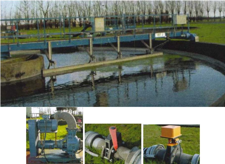
**Figure 7.12:** Pictures of the clarifier (top), the feed centrifugal pump (bottom left), the feed valve (bottom middle) and the recycle valve (bottom right) of the Heist WWTP
