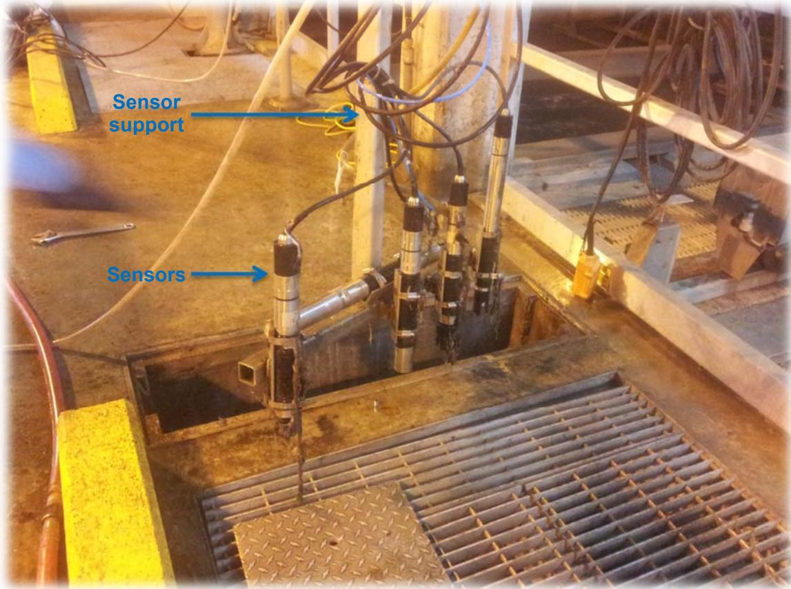
Figure 18: Entrance of grit chamber installation
