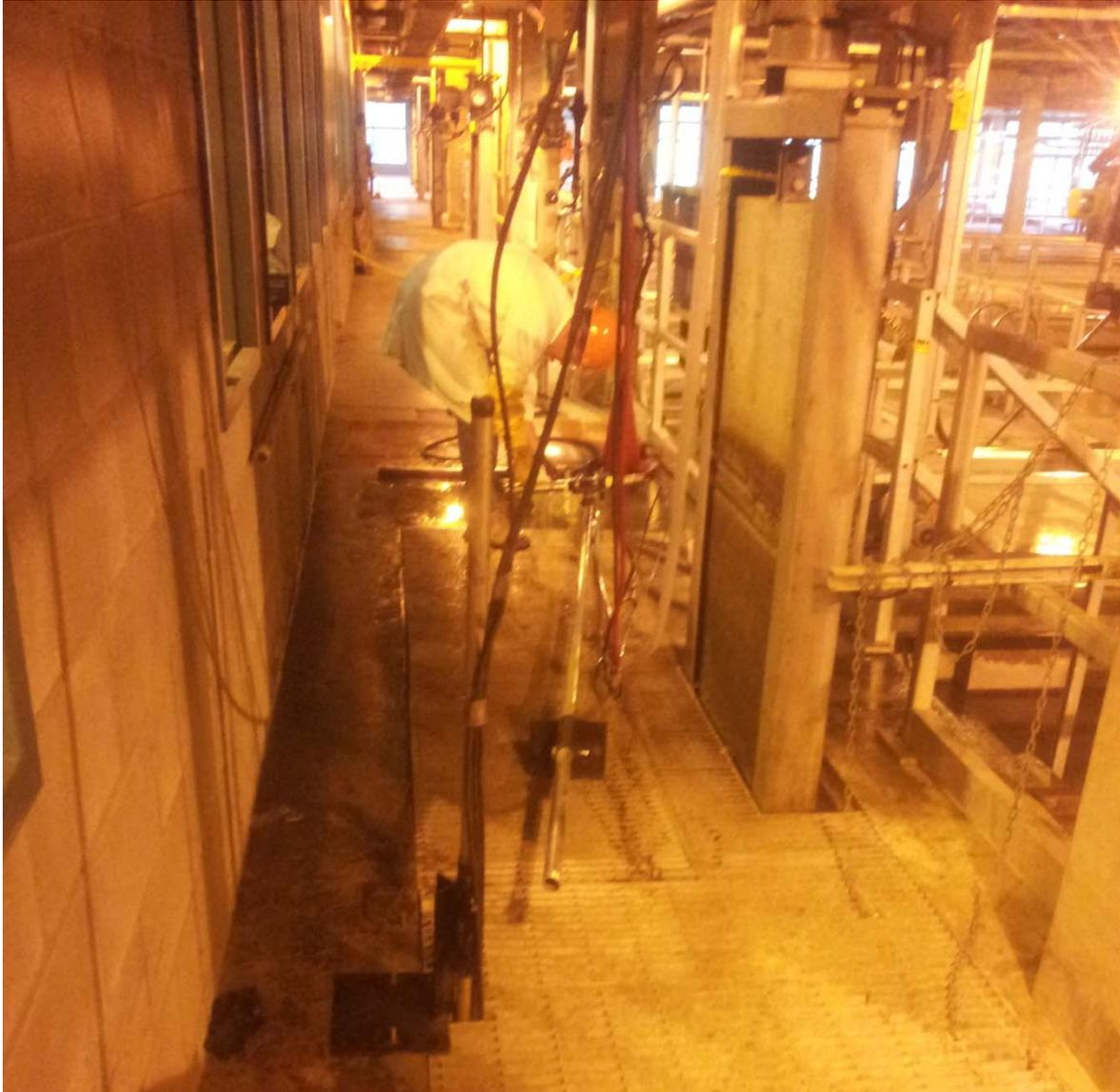
Figure 26: Cleaning sensors
