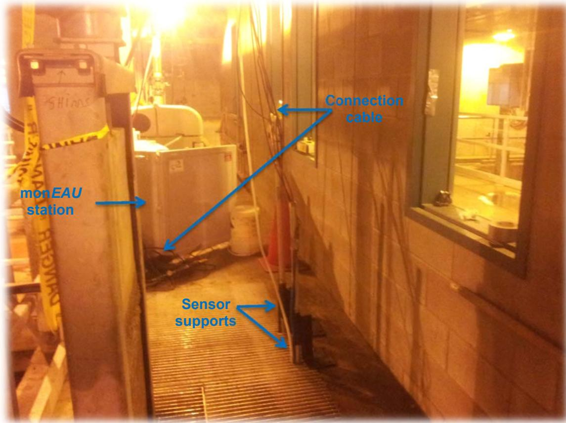
**Figure 14: Primary clarifier installation n°1**
