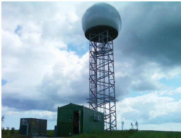
DMI's Viring radar in Denmark. Based on, for example, radar images a forecast of the precipitation can be made and used in the control of the wastewater system.
