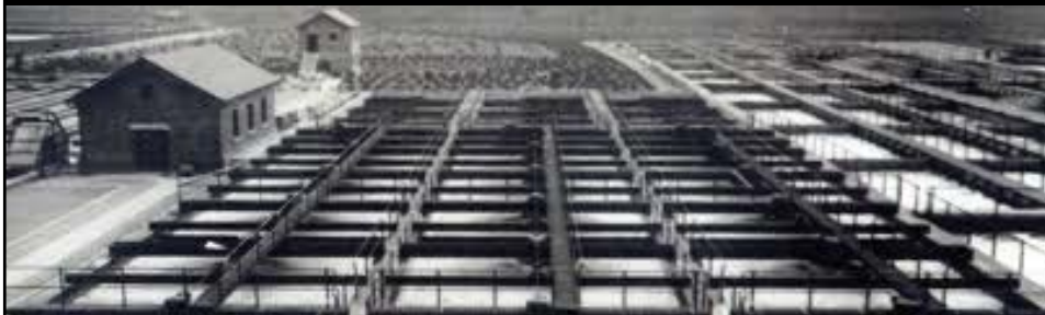
Davyhulme WWTP, Manchester, UK
